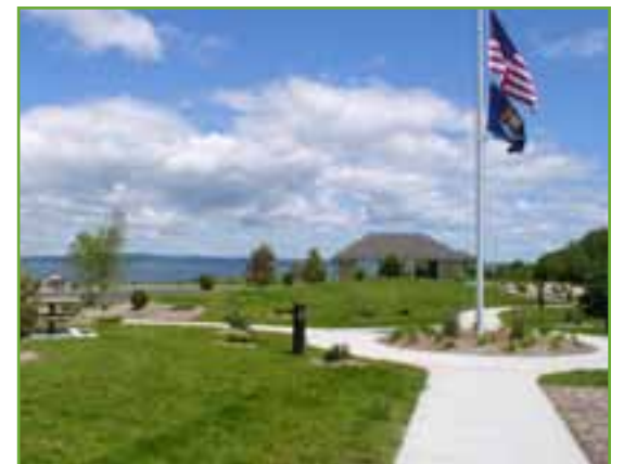
The work completed by CMS Land has provided additional environmental improvements to Little Traverse Bay.
